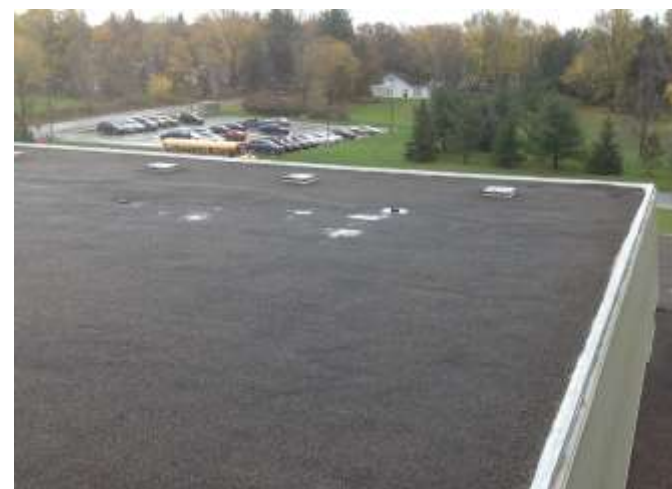
New Roof/ Restoration
